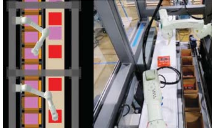
A side-by-side view of the K-ROSET cell simulation and the robots in production.
